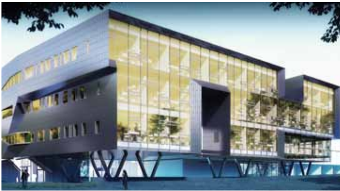
The Stephen Hawking Centre at Perimeter Institute
